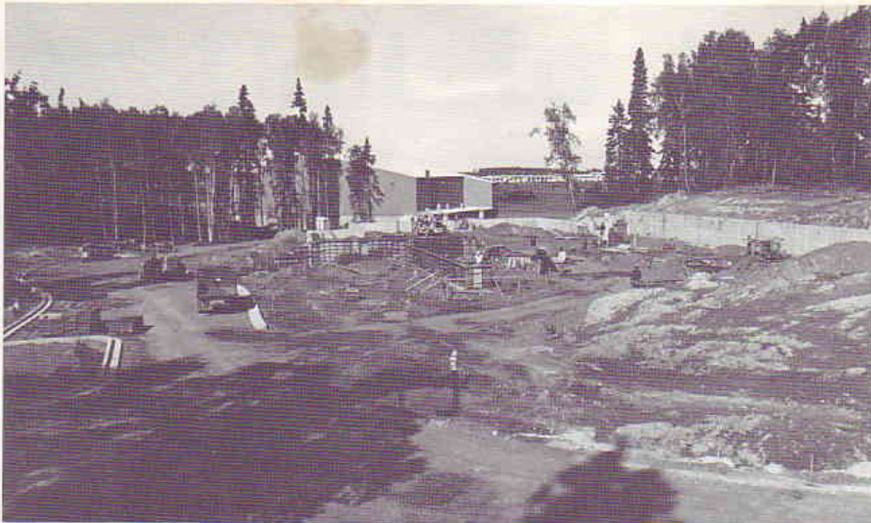
Laying the Foundation. Beginning to build the new Operations & Training Building at Kulis ANO Base. Jul. 1984.
