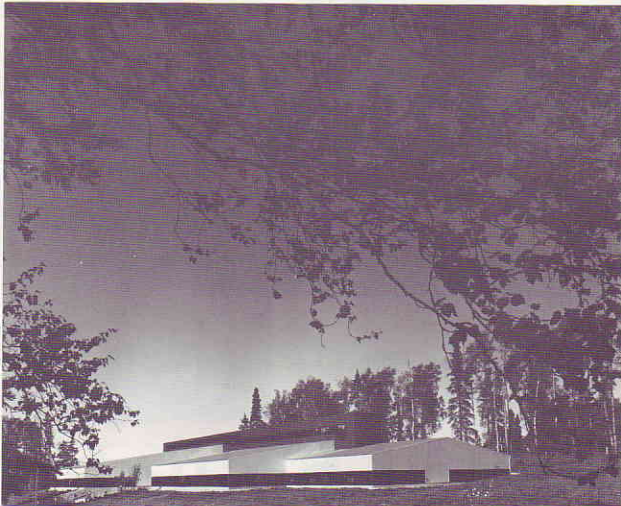
Finished O&T Building. winner of USAF Merit Award for Completed Project, then DOD's Blue Seal Award for Design Excellence. June 1985.
